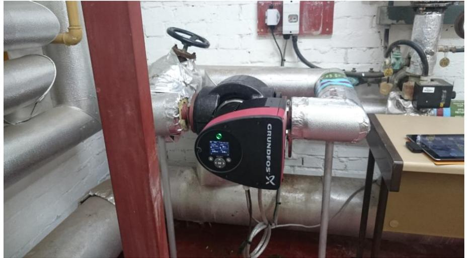
A recent installation with a Grundfos heating pump . This pump has been fitted with two temperature sensors to enable it to have a 10° differential set-point
