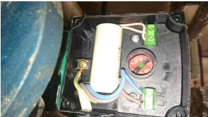
Flow monitoring was able to identify this pump fault on speed three thus enabling a temporary fix to get heat back in the building. The pump was later exchanged for a new self-regulating circulation pump
